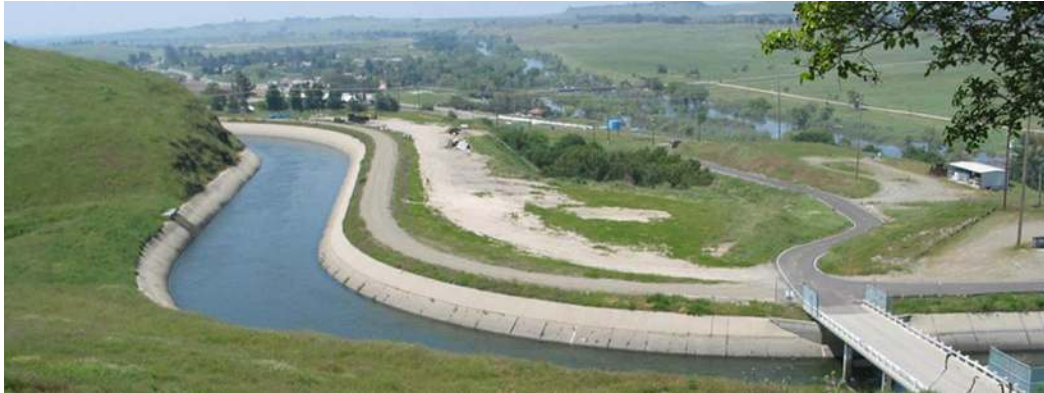
Figure 20.2.7: The California Aqueduct carries water needed for agriculture from Northern California to Southern California.
