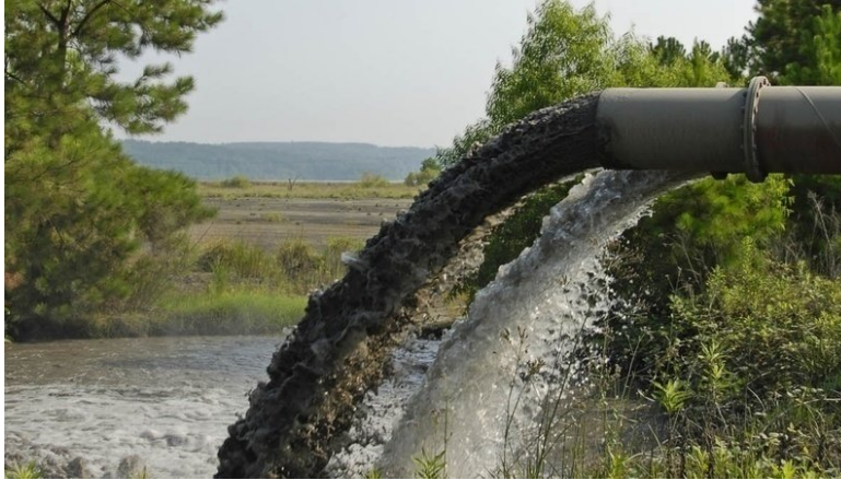
Figure 22.8 Photo of discharge of industrial waste into river
