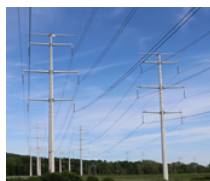
Figure 1.1.1 : 345,000 volt transmission lines.
