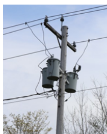
Figure 10.4.2 : A cluster of three residential power transformers.
