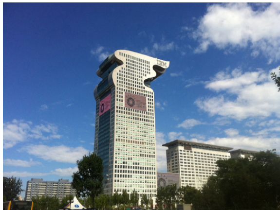
Exhibit 9.7 IBM building in China IBM is a U.S.-based company with several divisions organized geographically. Pictured here is the “Dragon Building,” their China-based headquarters. (Credit: bfishshadow/ flickr/ Attribution 2.0 Generic (CC BY 2.0))
