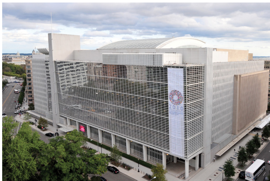
Figure 6.2 World Bank Headquarters in Washington, DC
