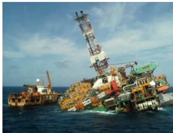
Figure 2.4.: The Petrobras P-36 oil platform sinking.
