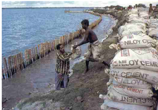
Figure 11.1.2: Bangladeshis Sandbagging Coastline. Source: "Environmental Geology of Developing Nations: Geology 351," Department of Geological Sciences, California State University, Los Angeles, accessed March 14, 2011, www.calstatela.edu/dept/geology/G351.htm .
