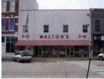
Figure 11.4.11: Tradition is important at Wal-Mart. Sam Walton's original Walton's Five and Dime is now the Wal-Mart Visitor's Center in Bentonville, Arkansas. Wikimedia Commons – CC BY-SA 2.5.
