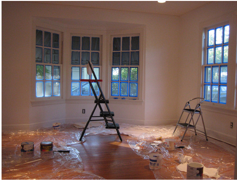
There are several distinct tasks involved in painting a room.
