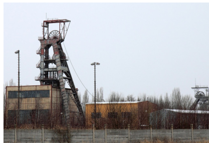
Figure 2.3.1: Coal is mined and moved by heavy machinery. The coal lift shown is 20th century and not modern. In Taylor's time, it was moved by shovel to rail cars or trucks. PublicDomainPictures – CC0 public domain.
