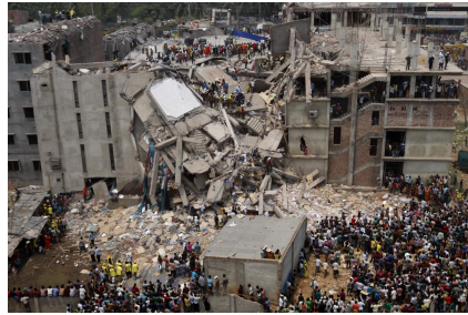
Figure 5.14.1: Garment factory collapse, Rana Plaza, Bangladesh.
