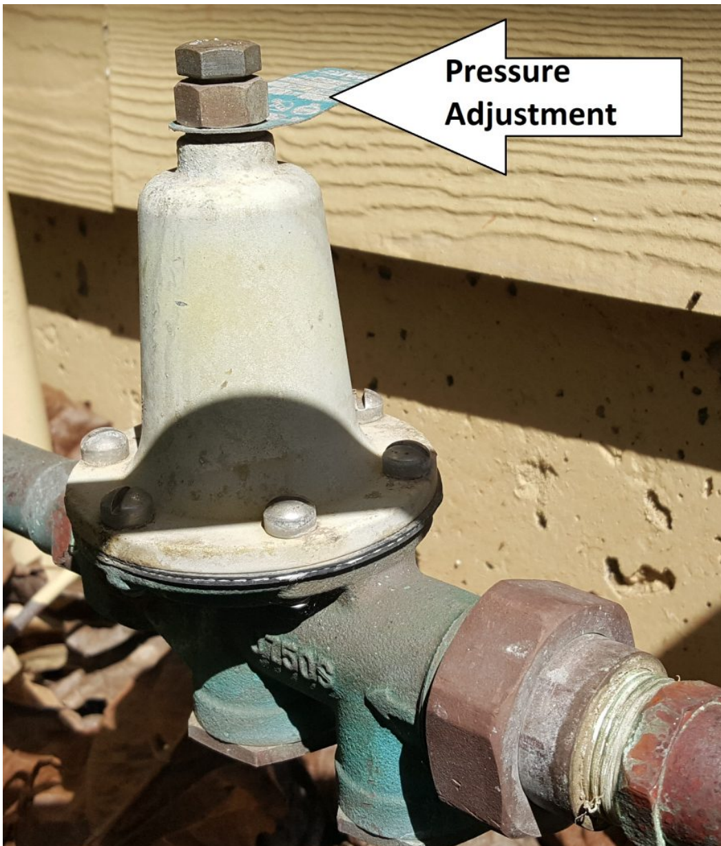
Pressure Regulator by Clifford Rutherford is licensed under CC BY 4.0
