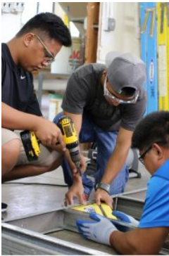
Figure 8.1.1: Construction Technology Program C3T Image 8366 is licensed under CC BY 4.0
