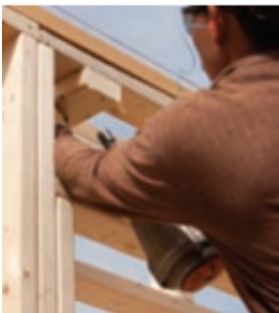
Nail penetration through the lumber is a special concern where the piece is held in place by hand. Nail gun by OSHA is licensed under Public Domain
