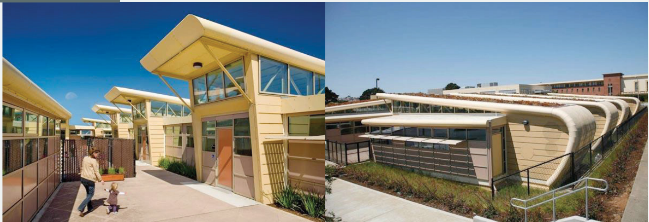
Figure 15.1.1: Project Frog Modules Linked to Make the Child Development Center, City College of San Francisco
