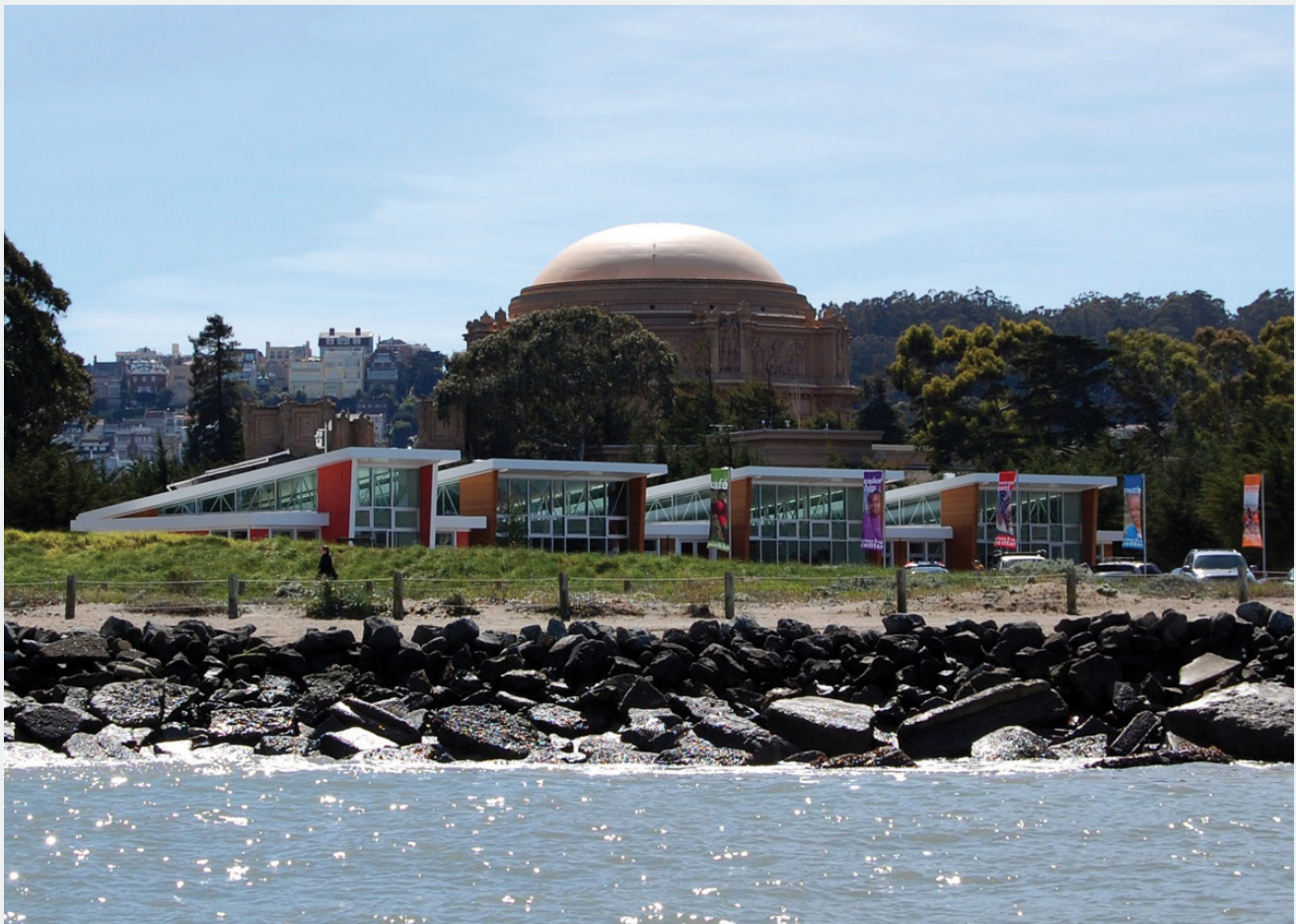
Figure 15.1.4: Crissy Field Center, San Francisco. Source: Project Frog. A virtual tour is at www.projectfrog.com/gallery/tour .
