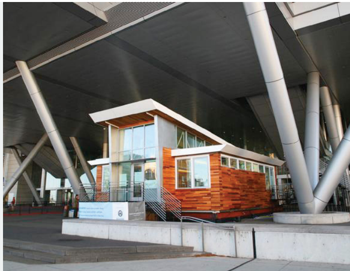
Figure 15.1.3: Exterior of Project Frog Zero at Greenbuild 2008. Source: Project Frog.
