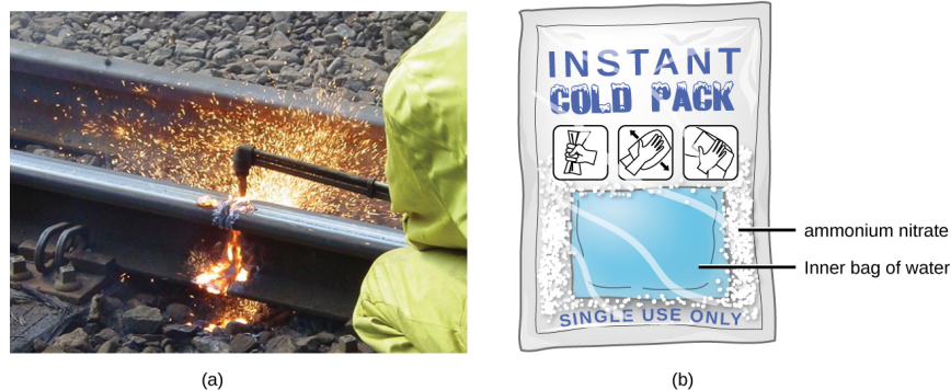
Figure 3: (a) An oxyacetylene torch produces heat by the combustion of acetylene in oxygen. The energy released by this exothermic reaction heats and then melts the metal being cut. The sparks are tiny bits of the molten metal flying away. (b) A cold pack uses an endothermic process to create the sensation of cold. (credit a: modification of work by “Skatebiker”/Wikimedia commons).
