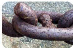
Figure 10.4.3: Rust (iron oxide) forms on an unprotected iron surface.
