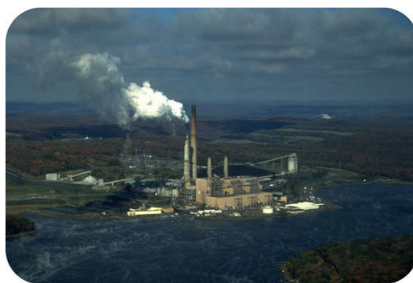
Figure 6.1.4: This power plant in West Virginia, like many others, is located next to a large lake so that the water from the lake can be used as a coolant. Cool water from the lake is pumped into the plant, while warmed water is pumped out of the plant and back into the lake.
