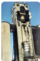
Figure 11.6.6: This grain elevator in Kansas exploded in 1998. The tiny size of the reacting particles (grain dust) caused the reaction with oxygen in the air to be violently explosive.
