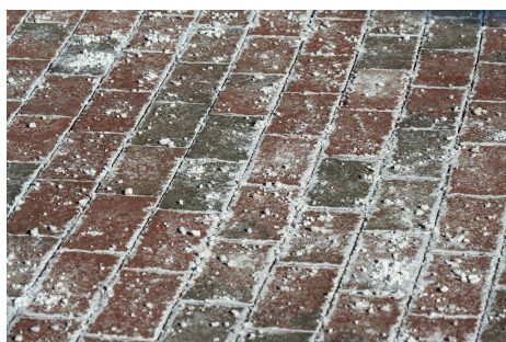
Figure 9.4.2: Effect of Freezing Point Depression. The salt sprinkled on this sidewalk makes the water on the sidewalk have a lower freezing point than pure water, so it does not freeze as easily. This makes walking on the sidewalk less hazardous in winter. © Thinkstock
