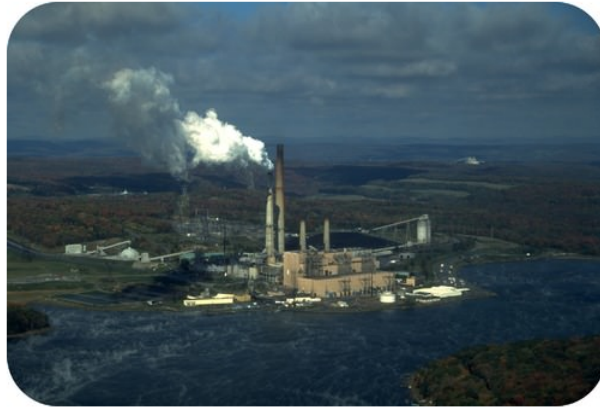
Figure 7.2.2: This power plant in West Virginia, like many others, is located next to a large lake so that the water from the lake can be used as a coolant. Cool water from the lake is pumped into the plant, while warmer water is pumped out of the plant and back into the lake.
