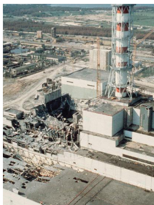
Figure 18.5.2 The Chernobyl Nuclear Power Plant In 1986, mechanical and operational failures during testing at the Chernobyl power plant in the USSR (now in the Ukraine) caused an uncontrolled nuclear chain reaction. The resulting fire destroyed much of the facility and severely damaged the core of the reactor, resulting in the release of large amounts of radiation that was spread over the surrounding area by the prevailing winds. The effects were devastating to the health of the population in the region and to the Soviet economy.
