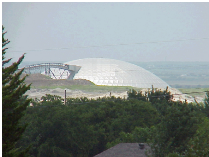
Figure 4.2.4.30: Exterior view of dome storage unit with conveyor loading port (Copyright Halliburton Energy Services).
