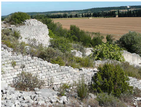
Figure 9.3.1: The Barbegal mill as it stands today.
