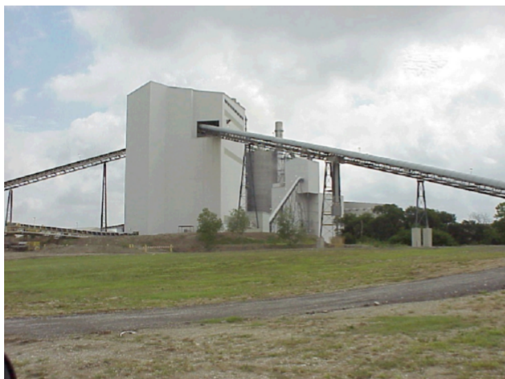
Figure 4.2.4.33: Buffer bin (Copyright Halliburton Energy Services).
