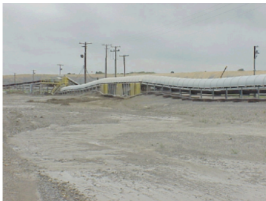
Figure 4.2.4.29: Covered conveyor belt for limestone transport (Copyright Halliburton Energy Services).
