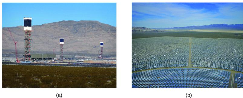
Figure 5.1.9: (a) The Ivanpah solar thermal plant uses 170,000 mirrors to concentrate sunlight on water-filled towers. (b) It covers 4000 acres of public land near the Mojave Desert and the California-Nevada border. (credit a: modification of work by Craig Dietrich; credit b: modification of work by "USFWS Pacific Southwest Region"/Flickr)
