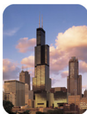
Figure 6.3.2: The Willis Tower (formerly called the Sears Tower) in Chicago was once the tallest building in the world and is still the tallest in the Western Hemisphere. The use of steel columns makes it possible to build taller, stronger, and lighter buildings.
