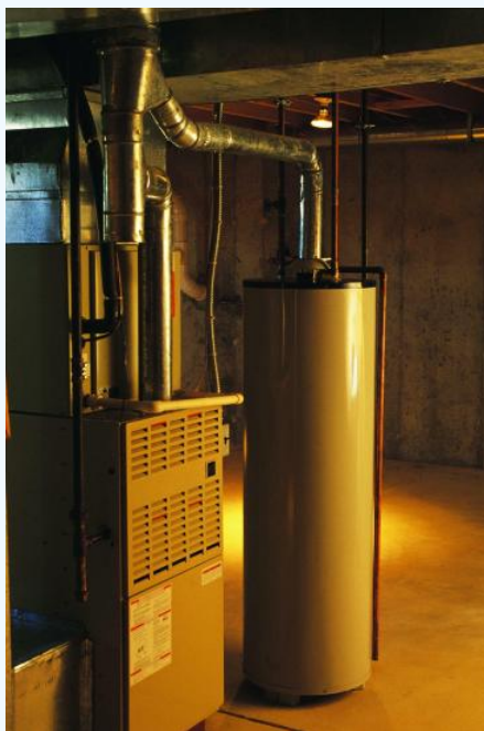
Figure 4.4.2 Tank water heater © Thinkstock. Most homes in the United States have a tank-type water heater like this one.
