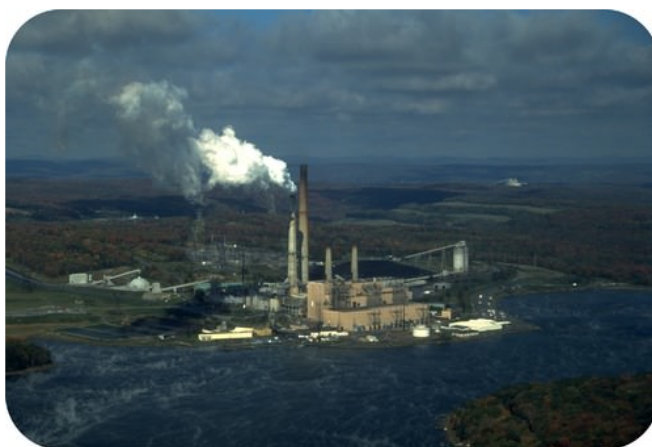
Figure 8.1.4 This power plant in West Virginia, like many others, is located next to a large lake so that the water from the lake can be used as a coolant. Cool water from the lake is pumped into the plant, while warmer water is pumped out of the plant and back into the lake.
