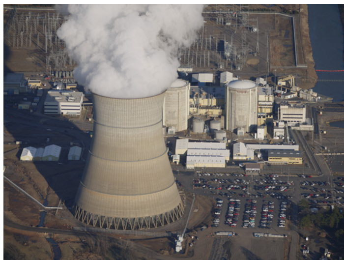
Figure 8.8.1: Russellville nuclear power plant in Arkansas, showing a cooling tower in the front with non-radioactive steam evaporating from it. Source: Edibobb, CC BY 3.0 < https://creativecommons.org/licenses/by/3.0 >, via Wikimedia Commons
