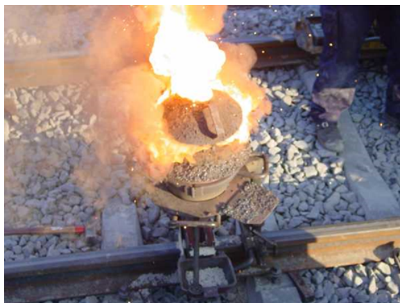
Figure 4.3.1: Thermite reaction proceeding. Shortly after this, the liquid iron flows into the mold around the rail gap. Source: http://en.Wikipedia.org/wiki/Image:V...ewelding-1.jpg , Public domain.
