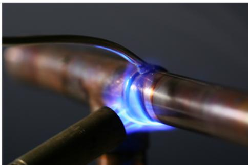
Figure 4.3.4: Propane torch being used to solder copper pipes for residential water mains. Source: Kevin L Neff / CC BY (<https://creativecommons.org/licenses/by/2.0>)
