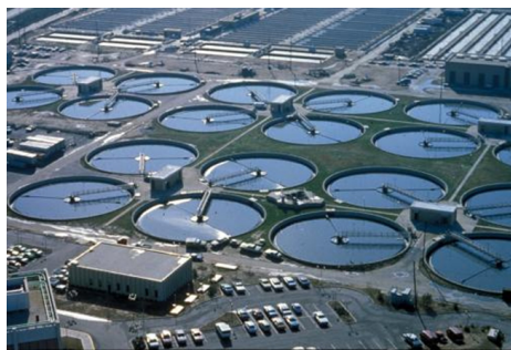
Figure 15.1.5: Wastewater treatment facilities, such as this one, remove contaminants from wastewater before the water is released back into the natural environment. (credit: "eutrophication&hypoxia"/Wikimedia Commons)
