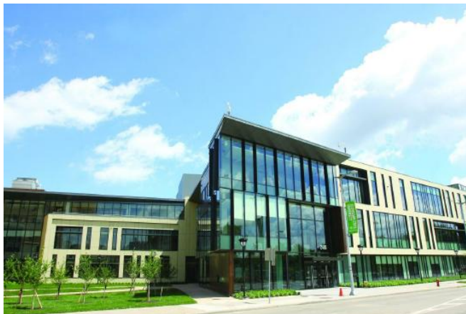
Figure [Math Processing Error] Outfitting a New Building. Source: Photo courtesy of Benjamin Benschneider, Cleveland State University.
