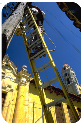
Figure 4.4.1 (Credit: Courtesy of the U.S. Department of Agriculture; Source: http://commons.wikimedia.org/wiki/File:Ladder_and_telegraph_pole.jpg (opens in new window); License: Public Domain)
