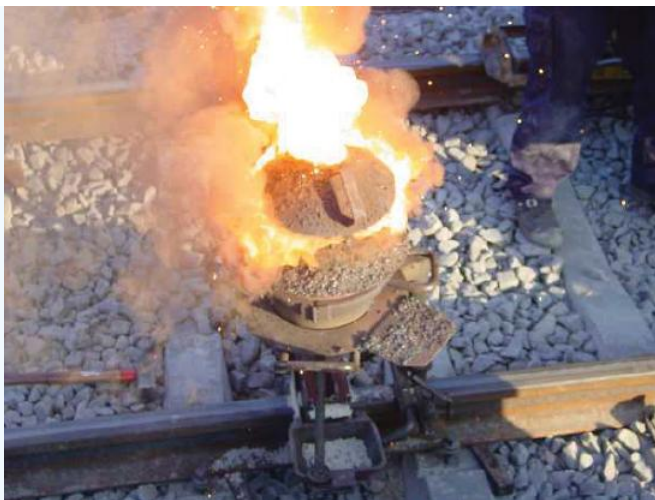
Figure 9.5.1 Thermite mixture. A small clay pot contains a thermite mixture. It is reacting at high temperature in the photo and will eventually produce molten metal to join the railroad tracks below it. (Public Domain; Skatebiker via Wikipedia )
