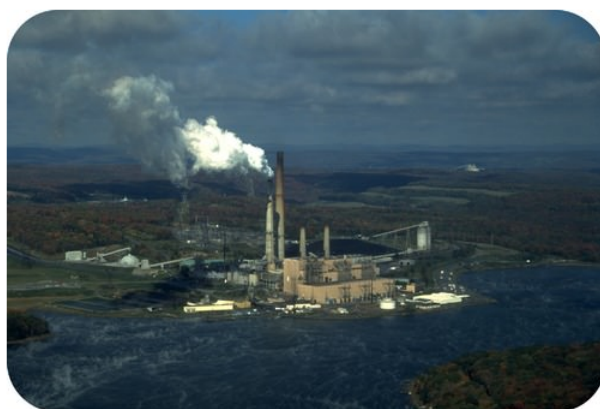
Figure 8.2.2: This power plant in West Virginia, like many others, is located next to a large lake so that the water from the lake can be used as a coolant. Cool water from the lake is pumped into the plant, while warmer water is pumped out of the plant and back into the lake.
