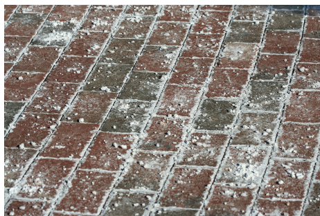
Figure 9.8.3: Effect of Freezing Point Depression. The salt sprinkled on this sidewalk makes the water on the sidewalk have a lower freezing point than pure water, so it does not freeze as easily. This makes walking on the sidewalk less hazardous in winter.
