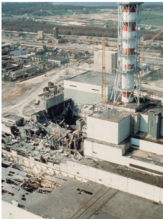
Figure 24.6.2: The Chernobyl Nuclear Power Plant. In 1986, mechanical and operational failures during testing at the Chernobyl power plant in the USSR (now in the Ukraine) caused an uncontrolled nuclear chain reaction. The resulting fire destroyed much of the facility and severely damaged the core of the reactor, resulting in the release of large amounts of radiation that was spread over the surrounding area by the prevailing winds. The effects were devastating to the health of the population in the region and to the Soviet economy.
