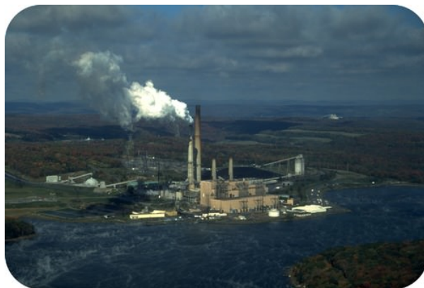
Figure 7.5.2.1: This power plant in West Virginia, like many others, is located next to a large lake so that the water from the lake can be used as a coolant. Cool water from the lake is pumped into the plant, while warmer water is pumped out of the plant and back into the lake.
