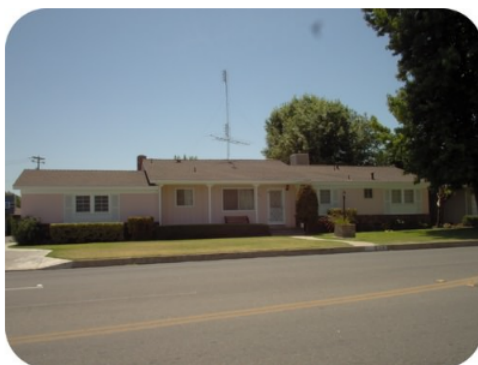
Figure 7.6.2.1: A home with a swamp cooler attached to the roof.
