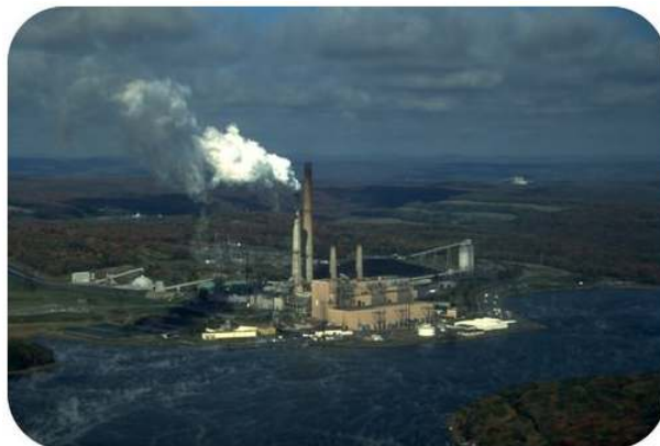
Figure 7.3.2: This power plant in West Virginia, like many others, is located next to a large lake so that the water from the lake can be used as a coolant. Cool water from the lake is pumped into the plant, while warmer water is pumped out of the plant and back into the lake.
