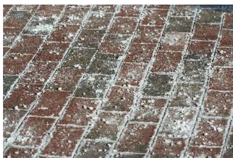
Figure 9.5.2: Effect of Freezing Point Depression. The salt sprinkled on this sidewalk makes the water on the sidewalk have a lower freezing point than pure water, so it does not freeze as easily. This makes walking on the sidewalk less hazardous in winter. © Thinkstock
