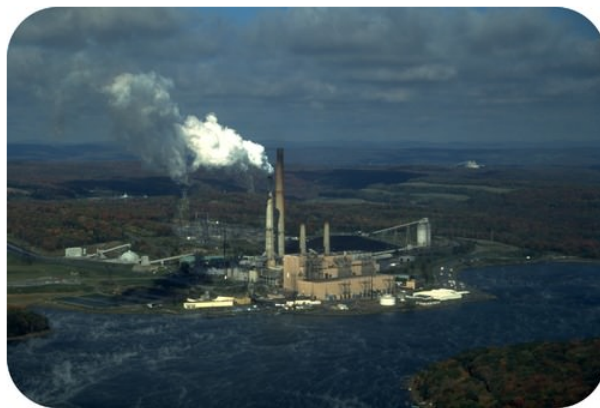
Figure 3.11.1: This power plant in West Virginia, like many others, is located next to a large lake so that the water from the lake can be used as a coolant. Cool water from the lake is pumped into the plant, while warmer water is pumped out of the plant and back into the lake.
