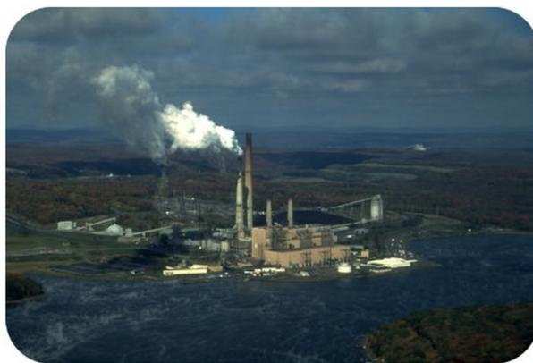
Figure 11.2.1: This power plant in West Virginia, like many others, is located next to a large lake so that the water from the lake can be used as a coolant. Cool water from the lake is pumped into the plant, while warmer water is pumped out of the plant and back into the lake.
