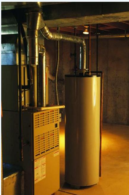
Figure 11.2.1.2 Tank water heater © Thinkstock. Most homes in the United States have a tank-type water heater like this one.
