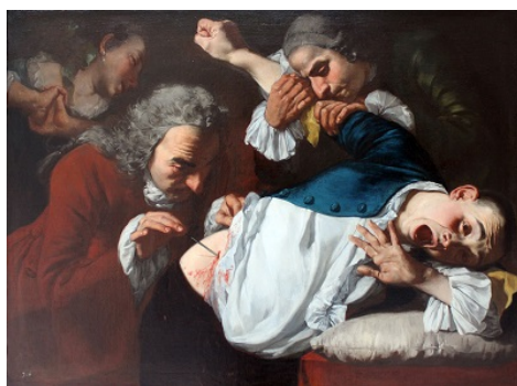
An operation in 1753, painted by Gaspare Traversi, of a surgery before antiseptics were used.
