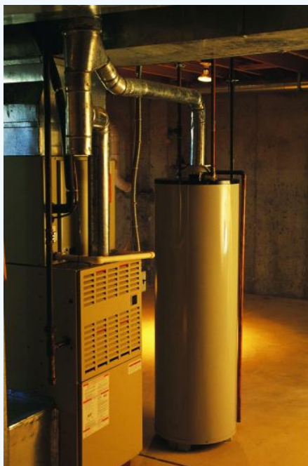
Figure 3.11.2 Tank water heater © Thinkstock. Most homes in the United States have a tank-type water heater like this one.
