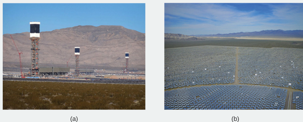
Figure 2.2.1.9: (a) The Ivanpah solar thermal plant uses 170,000 mirrors to concentrate sunlight on water-filled towers. (b) It covers 4000 acres of public land near the Mojave Desert and the California-Nevada border. (credit a: modification of work by Craig Dietrich; credit b: modification of work by “USFWS Pacific Southwest Region”/Flickr)
