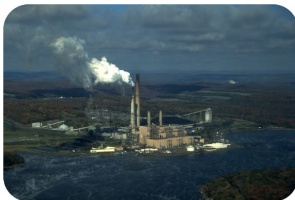
Figure 1.3.4.2.1 : This power plant in West Virginia, like many others, is located next to a large lake so that the water from the lake can be used as a coolant. Cool water from the lake is pumped into the plant, while warmer water is pumped out of the plant and back into the lake. (CC BY-NC; CK-12)
