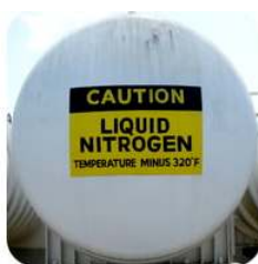
Figure 14.11.1: Nitrogen gas that has been cooled to 77 K has turned to a liquid and must be stored in a vacuum insulated container to prevent it from rapidly vaporizing. (CC BY-NC; CK-12)
