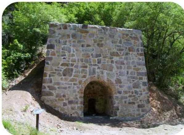
Figure 20.6.1: This lime kiln in Cornwall was used to produce quicklime (calcium oxide), an important ingredient in mortar and cement.
