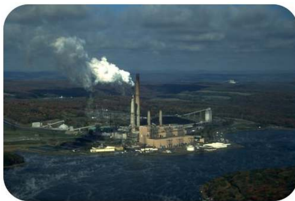
Figure 17.4.1: This power plant in West Virginia, like many others, is located next to a large lake so that the water from the lake can be used as a coolant. Cool water from the lake is pumped into the plant, while warmer water is pumped out of the plant and back into the lake. (CC BY-NC; CK-12)
