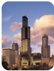
Figure 8.12.3: The Willis Tower (formerly called the Sears Tower) in Chicago was once the tallest building in the world, and is still the tallest in the Western Hemisphere. The use of steel columns makes it possible to build taller, stronger, and lighter buildings. (The copyright holder of this work allows anyone to use it for any purpose including unrestricted redistribution, commercial use, and modification; User:Soakologist/Wikipedia via Wikipedia )
