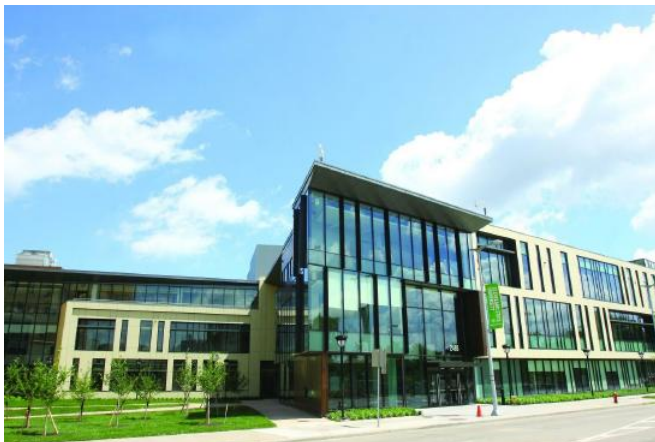
Figure 5.1.1 Outfitting a New Building. Source: Photo courtesy of Benjamin Benschneider, Cleveland State University.
