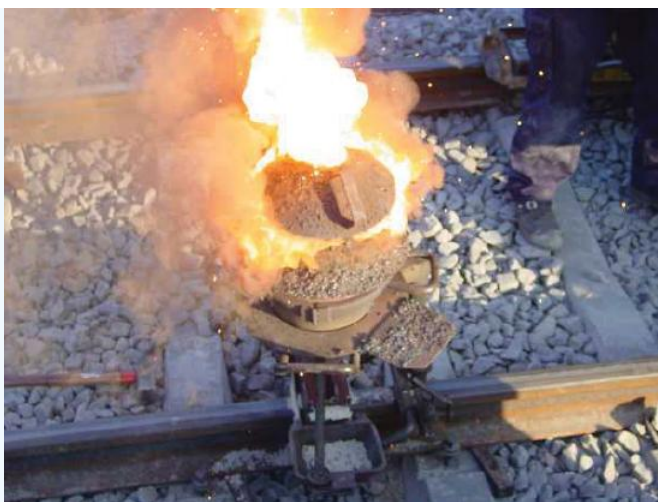
Figure 7.5.1 Thermite mixture. A small clay pot contains a thermite mixture. It is reacting at high temperature in the photo and will eventually produce molten metal to join the railroad tracks below it. (Public Domain; Skatebiker via Wikipedia )
