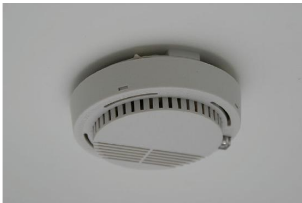
Figure 15.1.1: Smoke Detector. (CC SA -BY 3.0; Tumi-1983).
