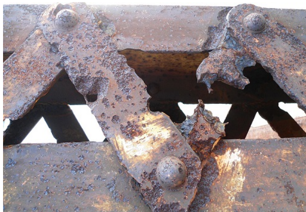
Figure 14.1.1: Corroded beams on the Nandu River Iron Bridge. These support beams on the bridge are obviously rusted. If the rusting becomes too bad, it will compromise the integrity of the bridge, requiring replacement. (Public Domain; Anna Frodesiak.)
