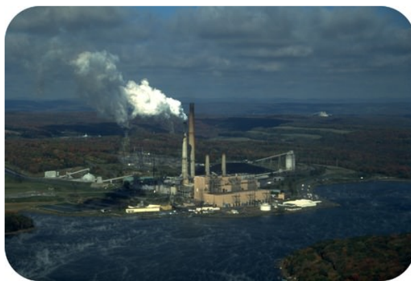
Figure 3.9.1: This power plant in West Virginia, like many others, is located next to a large lake so that the water from the lake can be used as a coolant. Cool water from the lake is pumped into the plant, while warmer water is pumped out of the plant and back into the lake.
