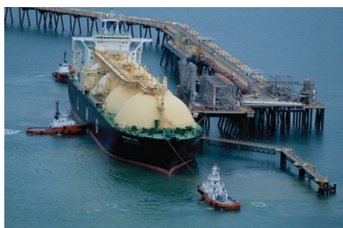
Figure 5.6.5: A Liquid Natural Gas Transport Ship.
