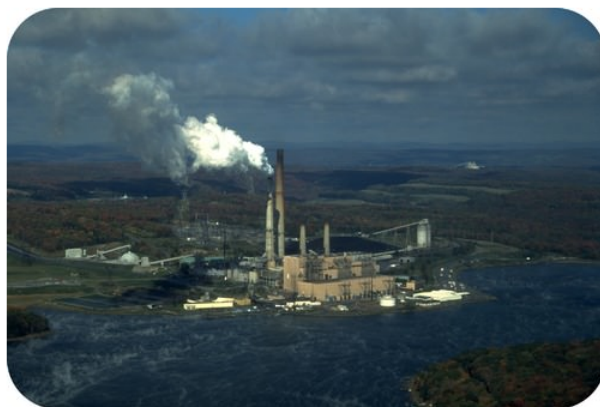
Figure 1.11.4: This power plant in West Virginia, like many others, is located next to a large lake so that the water from the lake can be used as a coolant. Cool water from the lake is pumped into the plant, while warmer water is pumped out of the plant and back into the lake.
