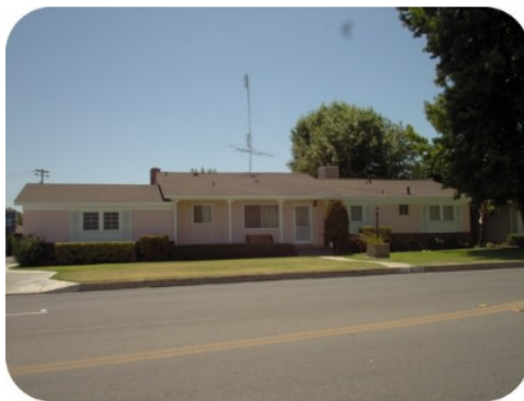
Figure 12.4.1: A home with a swamp cooler attached to the roof.
