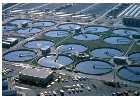
Figure 7.1.5: Wastewater treatment facilities, such as this one, remove contaminants from wastewater before the water is released back into the natural environment. (credit: “eutrophication&hypoxia”/Wikimedia Commons)
