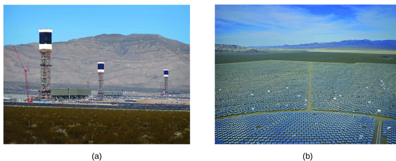
Figure 3.2.9: (a) The Ivanpah solar thermal plant uses 170,000 mirrors to concentrate sunlight on water-filled towers. (b) It covers 4000 acres of public land near the Mojave Desert and the California-Nevada border. (credit a: modification of work by Craig Dietrich; credit b: modification of work by "USFWS Pacific Southwest Region"/Flickr)
