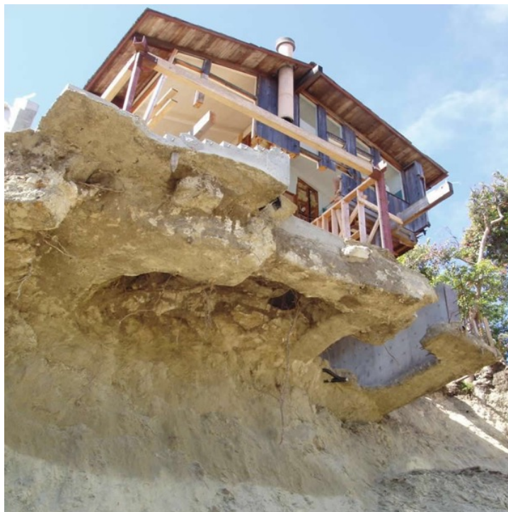
Figure 4. This photo shows one of the houses damaged by the 2005 Laguna Beach Landslide. The house experienced an undermining of the landslide but remained intact.
