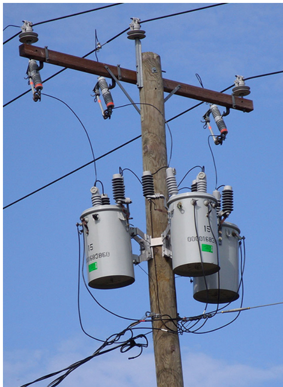
Figure 10.7.2: Transformers are used to step down the high voltages in transmission lines to the 110 to 220 V used in homes. (credit: modification of work by “Fortyseven”/Flickr)
