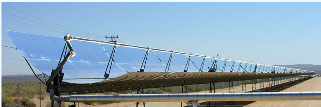
Figure 11.10.3.7: Parabolic trough collectors are used to generate electricity in southern California. (credit: "kjkolb"/Wikimedia Commons)
