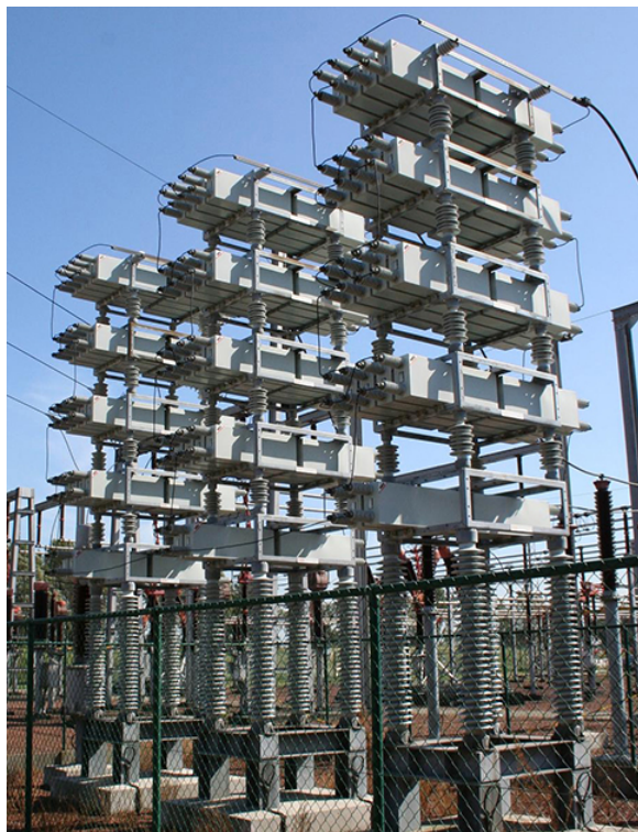
Figure 10.4.4: Power capacitors are used to balance the impedance of the effective inductance in transmission lines.
