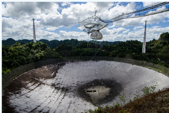
Figure 13.6.4: A 305-m-diameter paraboloid at Arecibo in Puerto Rico is lined with reflective material, making it into a radio telescope. It is the largest curved focusing dish in the world. Although D for Arecibo is much larger than for the Hubble Telescope, it detects radiation of a much longer wavelength and its diffraction limit is significantly poorer than Hubble's. The Arecibo telescope is still very useful, because important information is carried by radio waves that is not carried by visible light. (credit: Jeff Hitchcock)
