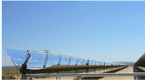
Figure [Math Processing Error]: Parabolic trough collectors are used to generate electricity in southern California. (credit: kjkolb, Wikimedia Commons)
