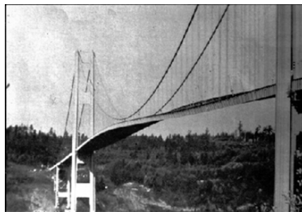
Figure 16.8.4: In 1940, the Tacoma Narrows Bridge in Washington state collapsed. Heavy cross winds drove the bridge into oscillations at its resonant frequency. Damping decreased when support cables broke loose and started to slip over the towers, allowing increasingly greater amplitudes until the structure failed (credit: PRI's Studio 360, via Flickr)
