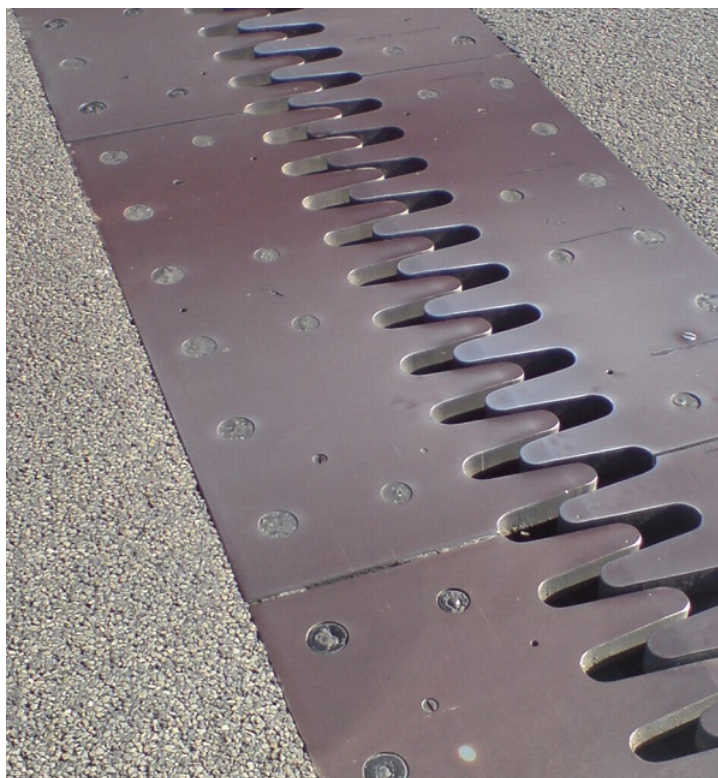
Figure 13.2.1: Thermal expansion joints like these in the Auckland Harbour Bridge in New Zealand allow bridges to change length without buckling. (credit: Ingolfson, Wikimedia Commons)
