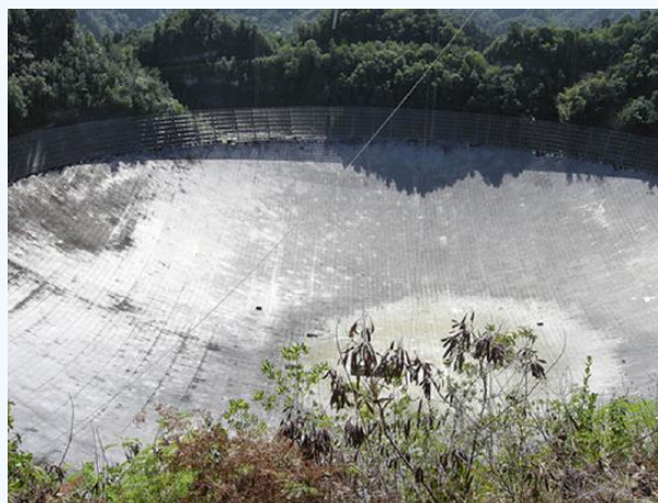
Figure 27.6.4: A 305-m-diameter natural bowl at Arecibo in Puerto Rico is lined with reflective material, making it into a radio telescope. It is the largest curved focusing dish in the world. Although D for Arecibo is much larger than for the Hubble Telescope, it detects much longer wavelength radiation and its diffraction limit is significantly poorer than Hubble's. Arecibo is still very useful, because important information is carried by radio waves that is not carried by visible light. (credit: Tatyana Temirbulatova, Flickr)
