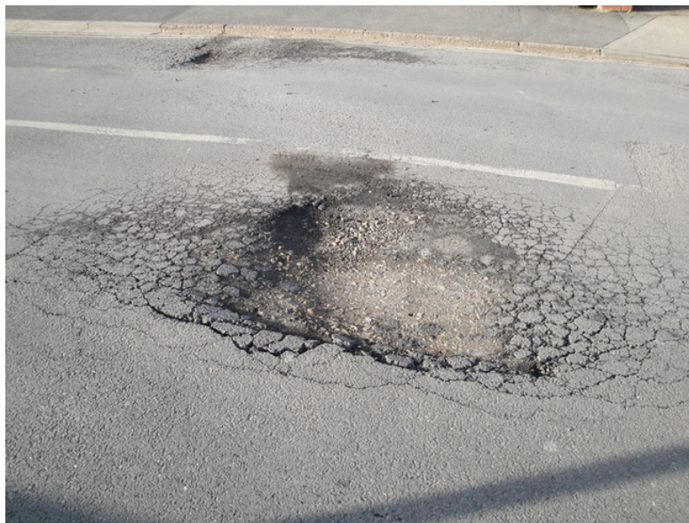
Figure 13.2.5: Thermal stress contributes to the formation of potholes. (credit: Editor5807, Wikimedia Commons)
