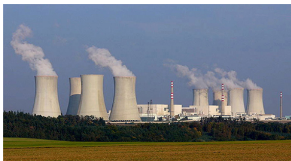
Figure 14.13.2: The heat exhausted from a nuclear power plant goes to the cooling towers, where it is released into the atmosphere.
