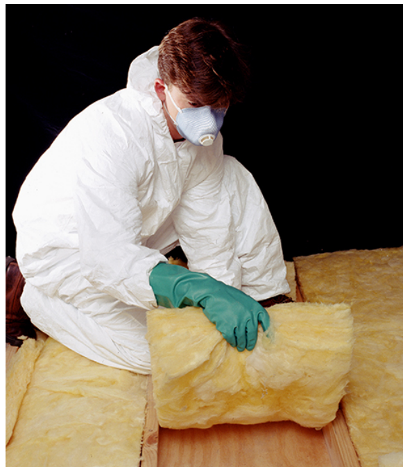
Figure 5: The fiberglass batt is used for insulation of walls and ceilings to prevent heat transfer between the inside of the building and the outside environment. (credit: Tracey Nicholls)
