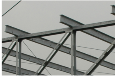
Figure 10.4.4: Steel I-beams are used in construction to reduce bending strains. (credit: modification of work by “US Army Corps of Engineers Europe District”/Flickr)
